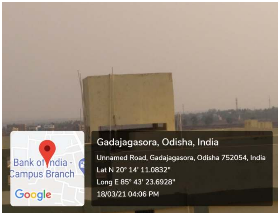
(Water Tank at the roof top in Academic Block)
