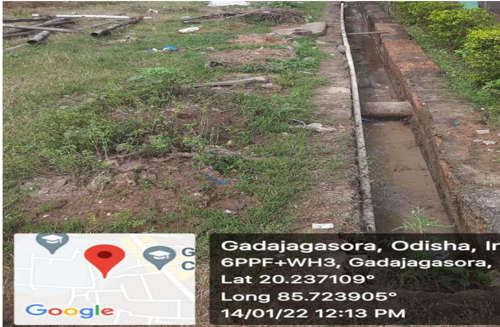
(Construction of bunds)
